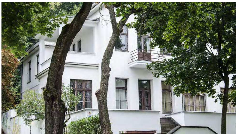
Figură 6. Centrul cultural Casa Artistului Kaunas, imagine: http://en.kaunas.lt/news/facade-repair-works-of-kaunas-artists-house
